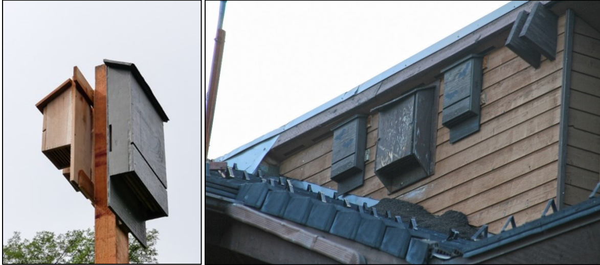
Figure 1. A bat box is a small type of bat house. A. A bat box is a small wooden box, often subdivided inside as “roosting chambers.” The extension of wood below the box is a landing platform where bats land, and then using their claws, they climb on the roughened wood up into the box. This particular installation has 2 bat boxes mounted on opposite sides of a pole; photo by J. Saremba. B. Bat boxes installed in an “array” on a building wall; photo by C. Olson.
