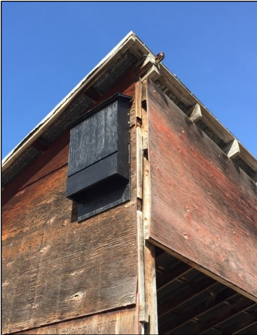
Figure 10. Standard four-chambered nursery box (BCI design – Photo by C. Olson).
