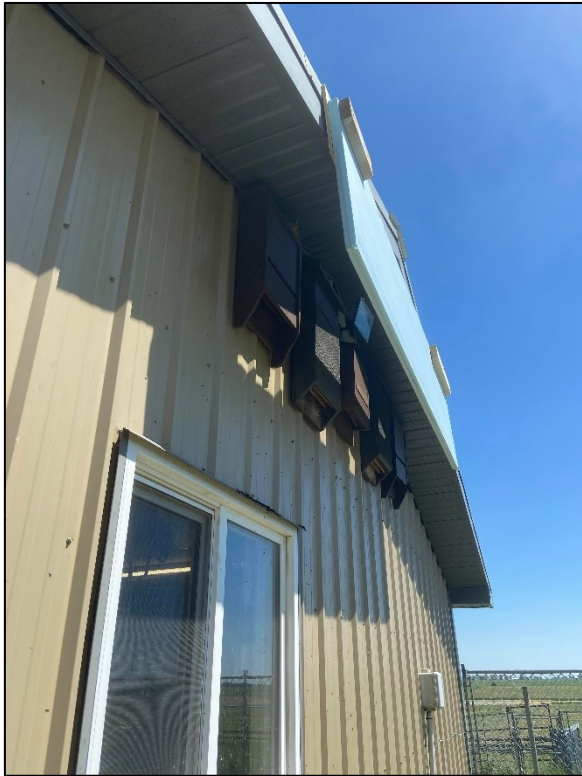
Figure 18. Landowner-installed sunshade -- insulated foam board attached to roof flashing as a temporary sunshade to protect bats during an extreme heat event. Photo by J. Thomson.
