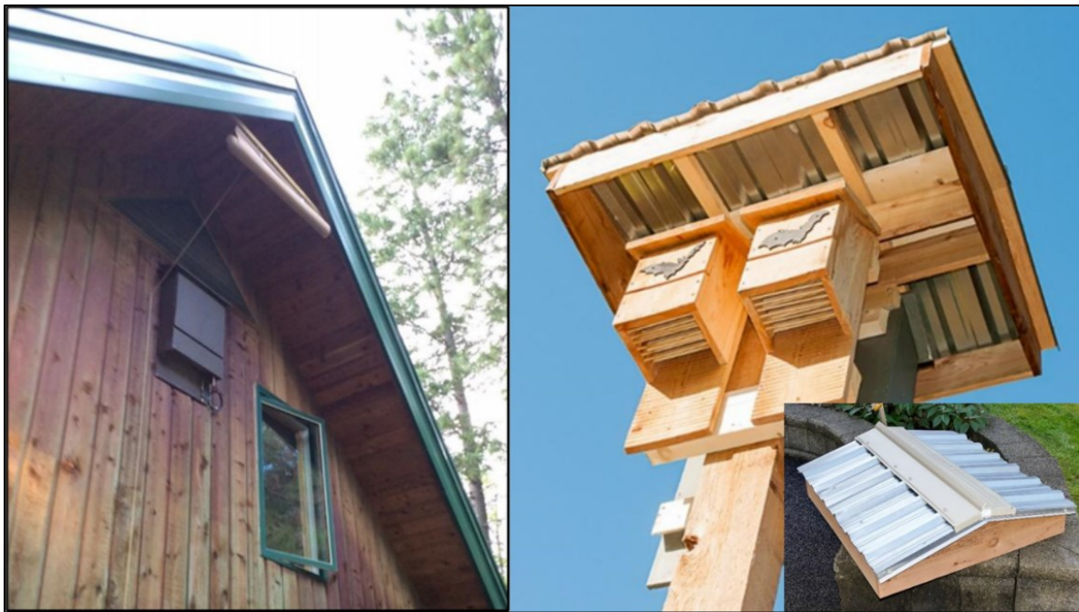
Figure 15. Two types of awnings. A. A rollup blind shade that is manually released via string (seen by bat box, extending to ground) with shade being applied by landowner only during periods of high heat (photo by Susan Dulc, design by Steve Latour, BC). B. A permanent awning designed to cast shade on bat boxes when the sun is highest in the sky; inset shows top of awning (photo and design by J. Saremba).
